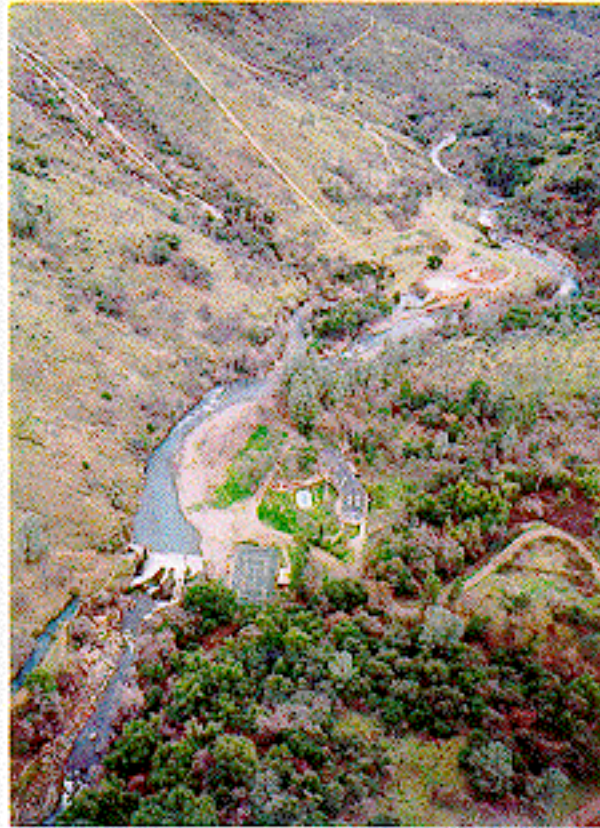
Photograph 3: Aerial view looking east at Inskip Diversion Dam on Battle Creek. South Powerhouse is located upstream, and the Oasis Springs Resort is located southeast of the diversion dam. (credit CDFG)
