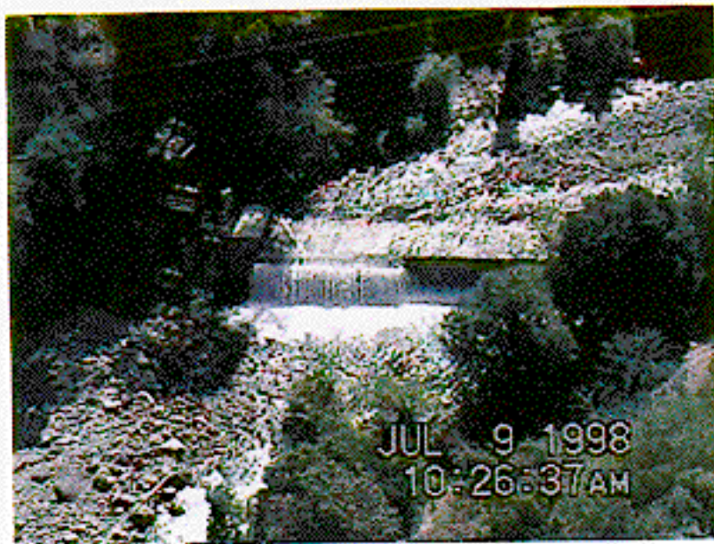
Photograph 6: View of downstream face of South Diversion Dam. (credit CDFG)
