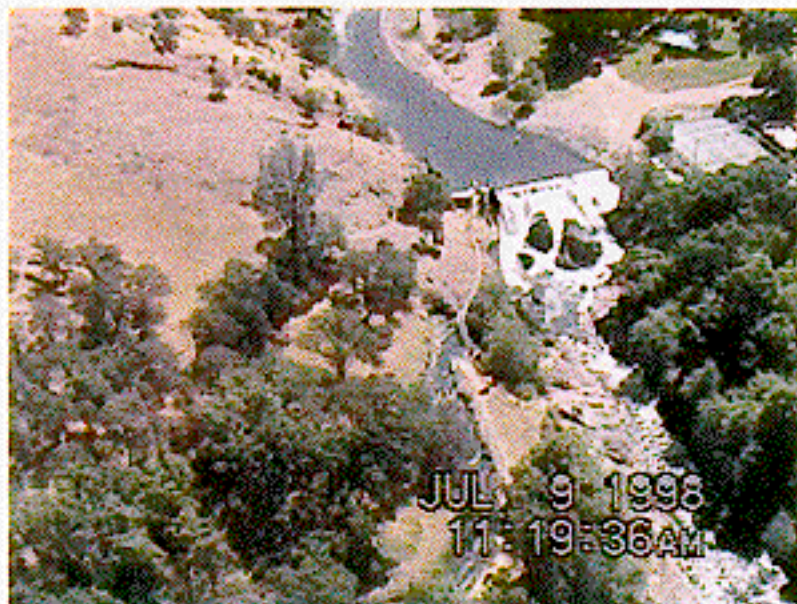
Photograph 4: Aerial view looking at downstream face of Inskip Diversion Dam. Note the large rocks that are present below the dam. (credit CDFG)
