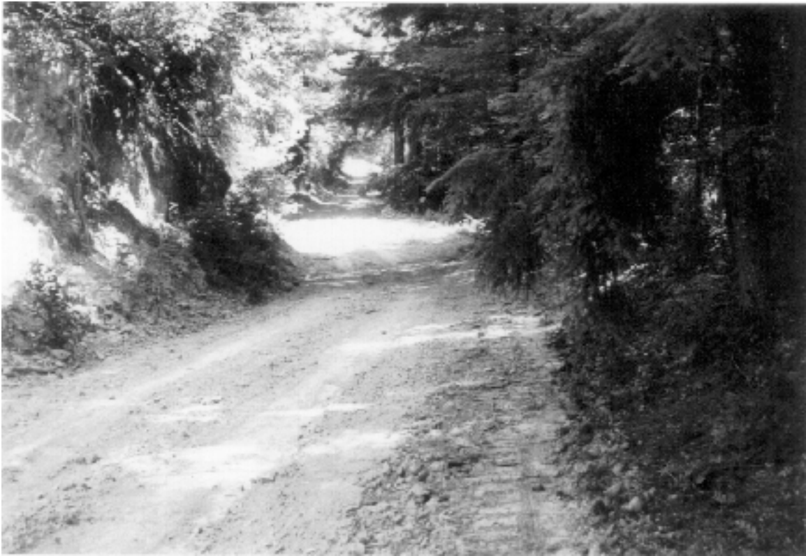
Figure 3. Site 13, B-Line. View looking down the road before erosion control efforts. The road bed in the middle portion of the photo between the cutbank and the twin redwoods in the distance has been constructed in a class 2 stream bed.
