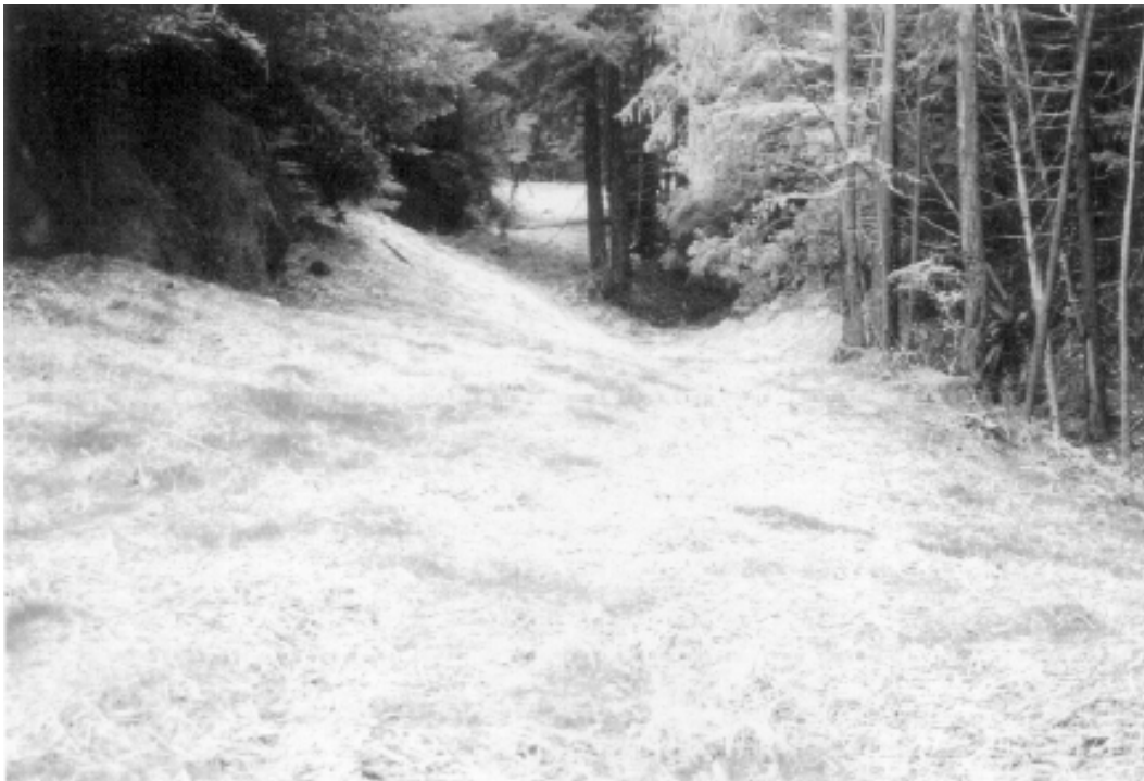
Figure 4. Site 13, B-Line. After treatment photo taken from the same location. The road bed has been decommissioned through this reach and a new 1000 foot section of no impact road has been constructed (not shown in the photo) to bypass this reach of road. The road was "put-to-bed" by excavating sidecast fill and outsloping the road. In the middle portion of the photo natural stream channel capacity has been re-established.
