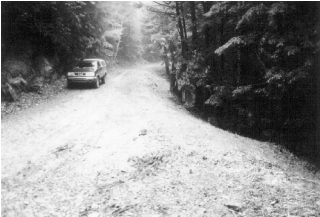
Figure 12. Site 106, G-005-01 Road. This after photograph exhibits the same treatment as in Figure 11 (i.e. excavating unstable fill material along the outside edge of the road), except for the road was not decommissioned but retained for future use. The fill material was excavated and loaded into dump trucks to be hauled to a stable location down the road for permanent storage. In upgrading the road, the road width was lessened, the inboard ditch was filled and eliminated, the road was re-shaped to exhibit a mild outslope with no berms, and periodic rolling dips were constructed along the road bed to ensure dispersed road runoff. Note the rolling dip about 60 feet behind the truck.
