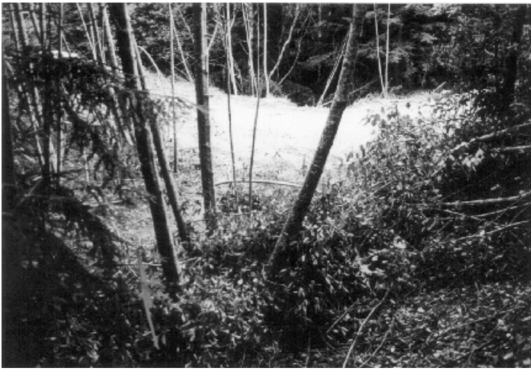
Figure 9. Site 100, G-005-01 Road. Before photo looking downstream at a large stream crossing to be decommissioned or properly pulled. Prior to opening the road to vehicular access, the road was completely overgrown with similarly sized alder as is visible in the photo. The crossing fill was eroding annual as a result of a plugged culvert. Future erosion at the site was estimated to be 525 yds 3 .
