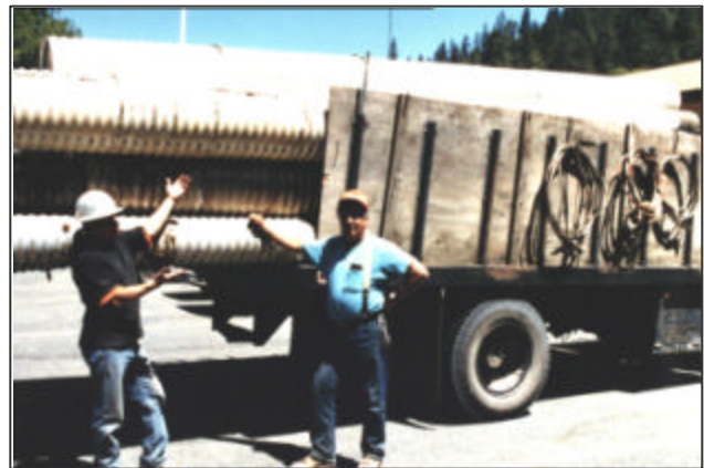
Culvert downspout being removed from the project.
