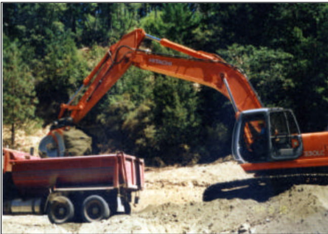
Excavator loading dump truck at RX10
