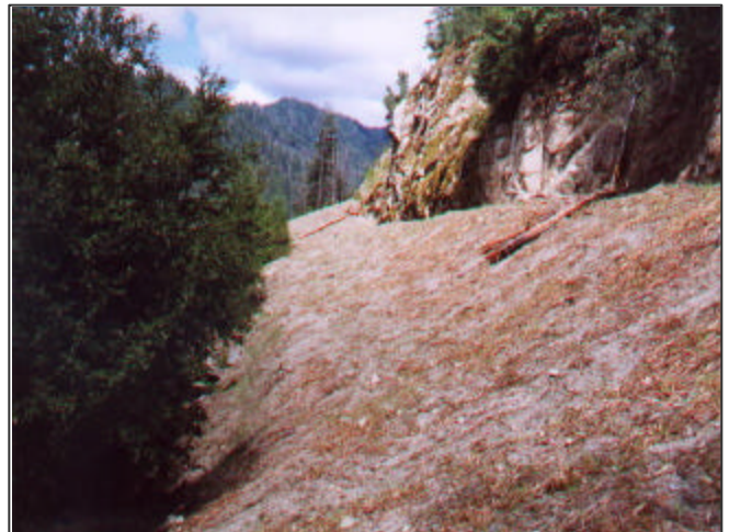
Photo point after outsliping imported fill.
