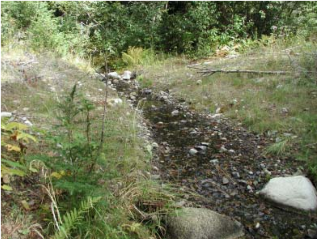
Reclaimed stream crossing on “old” Road 311.
