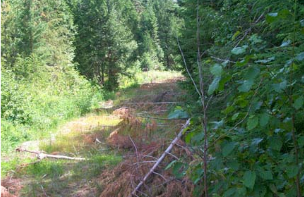
Photo showing obliterated portion of Road 312. This portion was hand-seeded over snow.
