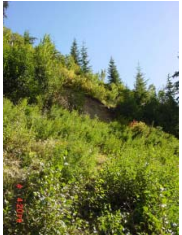
Pic. 6 – 1082D Cochran's Draw X-ing cut bank failure
