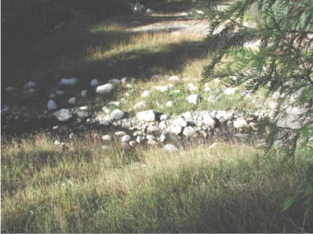
Cache Creek crossing on the “old” 311 road. On the earlier reviews in 1993, this crossing was considered a fish block. This restoration effort removed the fish block.
