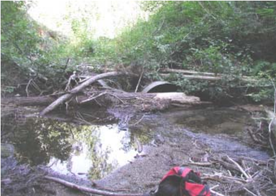
Inlet of culvert on Spread Creek under what was Road 1013.
