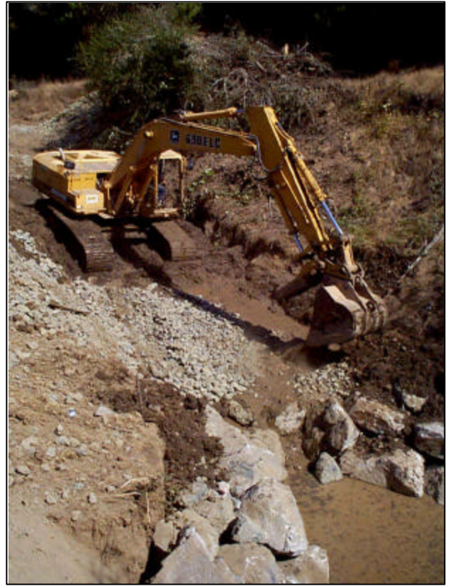
← Boulder Weir Installation ↑
