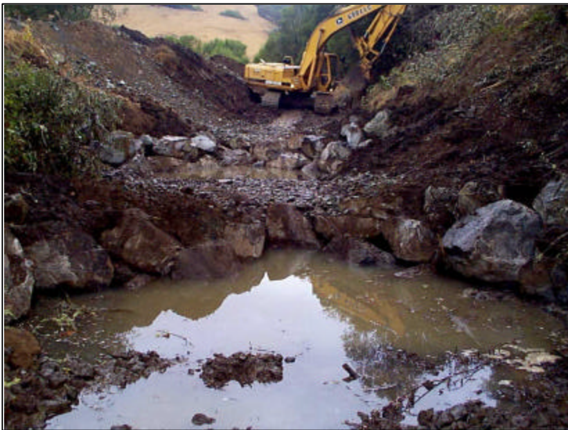
← Boulder Weir Installation ↑
