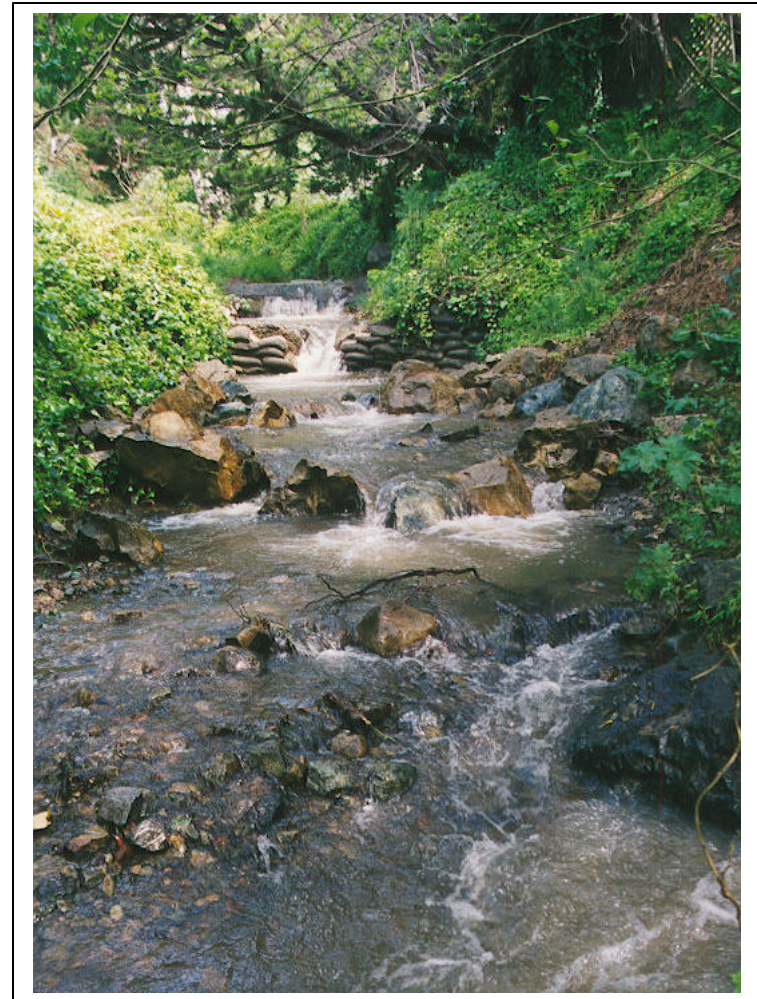
Figure 31: Photo (at left) looking upstream Laurel Creek at sacrete weir and grout structure just prior to construction (September 12, 1998) and photo (at right) looking upstream post-construction (1999) at created step-pools.
