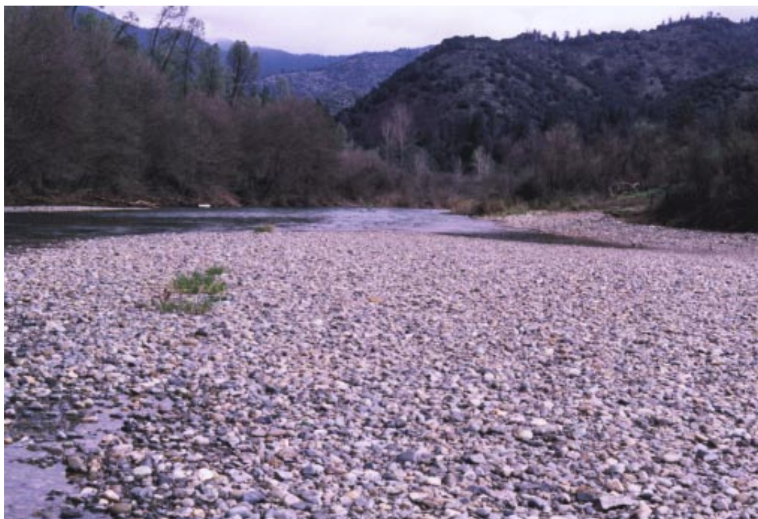
Figure 10.11 Sheridan Creek site after the 1995 flood. Note the large bar that developed along the constructed bank and the bar along the opposite bank. Some remnants of the original cobbles can be seen along the right edge of the photo. The grass growing from the bar (left of center) was grass that had established itself on the sediment retention berm shown in figure 10.52.
