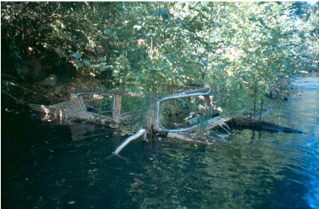
Figure 8: Ukiah Reach, Segment U4. This segment contained primarily flatwater habitat with well-developed riparian vegetation (top). Also, typical in this reach are past erosion control attempts that included lining the banks with automobile bodies (bottom).
